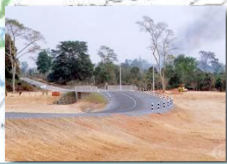
Bridge on Route 13 Rehabilitation (Grant)
