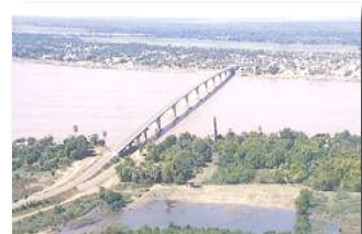
KIZUNA Bridge & National Road No.6-7 (Grant)
