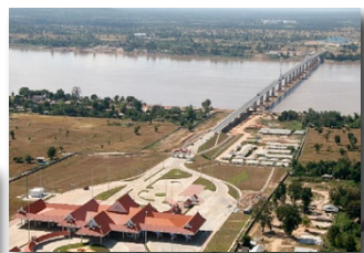
2nd Mekong International Bridge (Loan)
